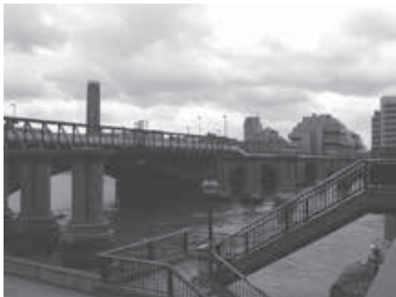
Blackfriars Bridge taken by the author
