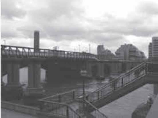
Blackfriars Bridge taken by the author
